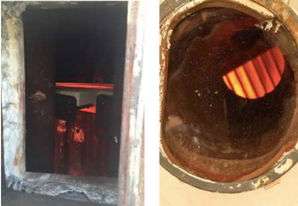
Figure 6. DUPLEX surface glow: view from viewing port on furnace shell (left), and view from viewing port on furnace floor (right). The surface glow may be considered a qualitative measure of performance, where a relatively uniform glow indicates good distribution of fuel and air along the surface, leading to optimal \text{NO}_x performance.
