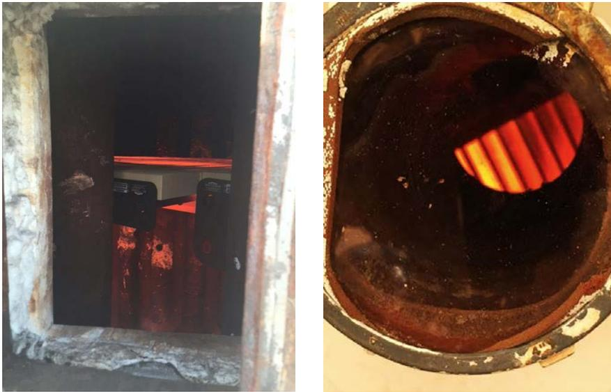
**Visible surface glow through viewing ports** located on the furnace shell (left) and floor (right) following the retrofit showed improved radiant heat transfer (Fig. 9).
