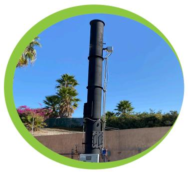
Complete flare systems include the flare tube, fuel skid, burner management system, and flame safeguards. Gas heating values ranging from 500 - 2,000 Btu/scf.
