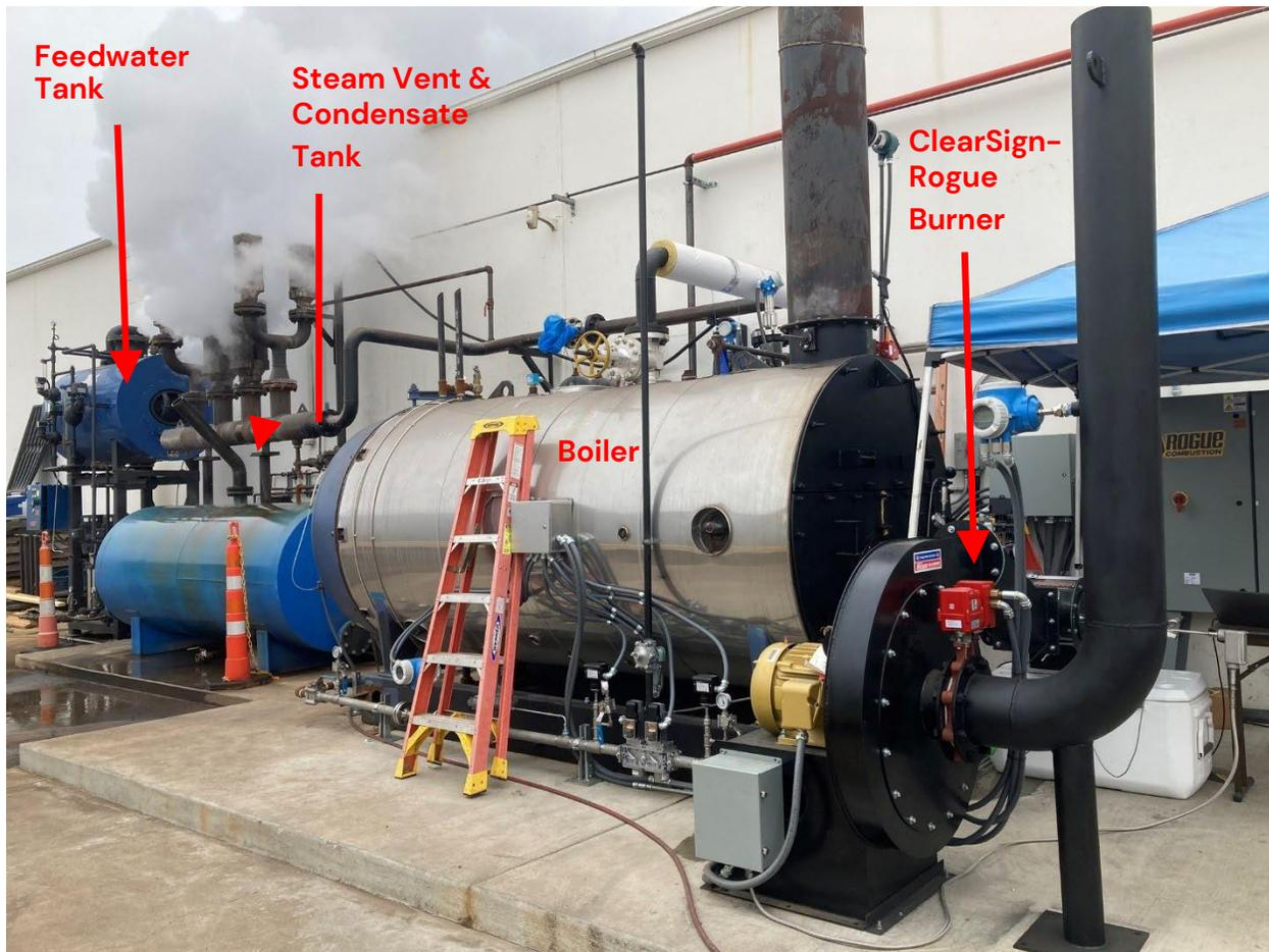
**Figure 7. Phase II Boiler Test Pad**
