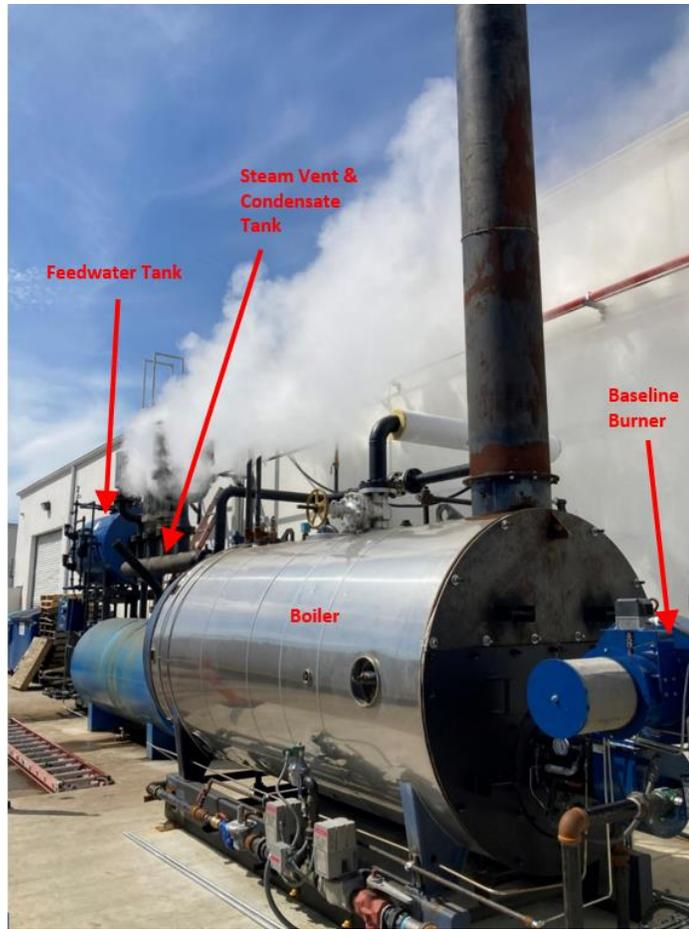
Figure 2. Boiler Test Pad Set-Up
