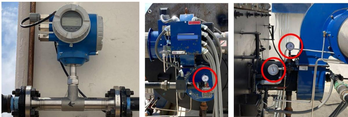
Figure 5. Burner Fuel Flow, Temperature, Pressure, and Combustion Air Pressure and Temperature Measurements.
