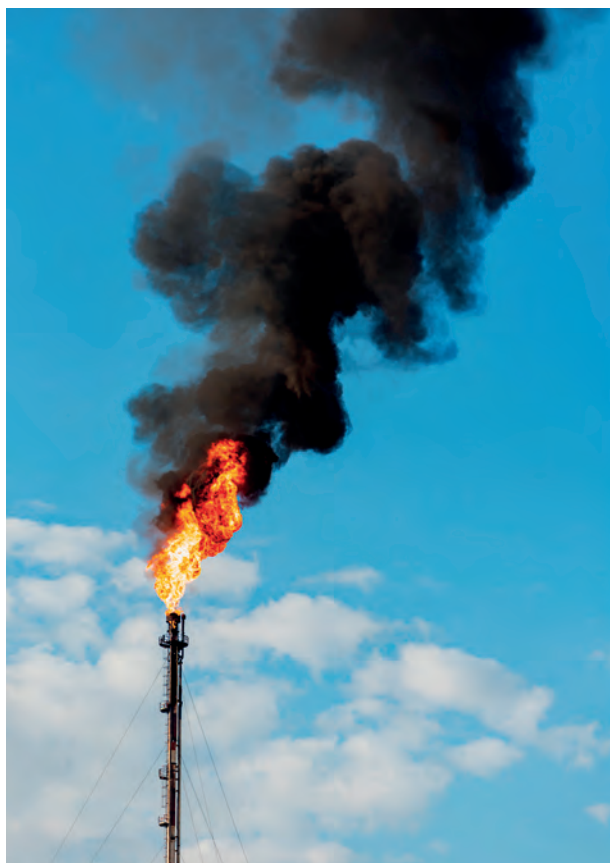
Figure 1. A elevated pipe flare in operation.
